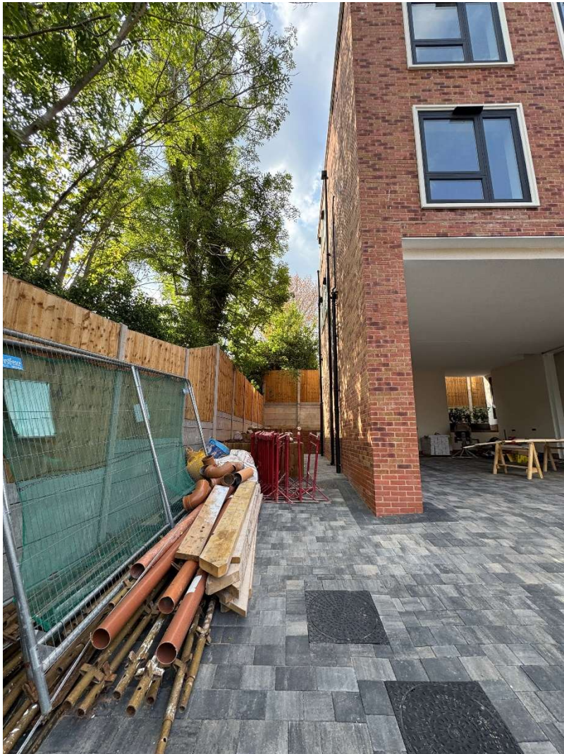
High level timber feather edge fencing on three and a half levels of concrete fence panels in front of existing palisade fencing on the railway border.
