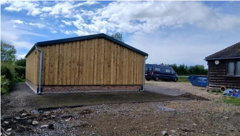
Image 2: Photograph of the East Elevation.
