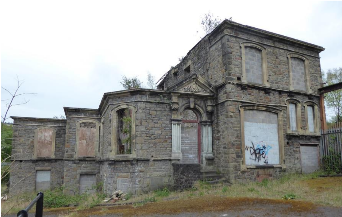
View of Laboratory Building prior to refurbishment works taking place.
